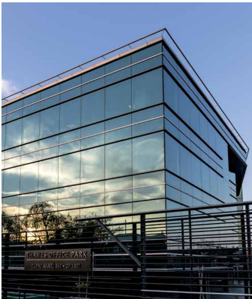
THAMES OFFICE PARK.
