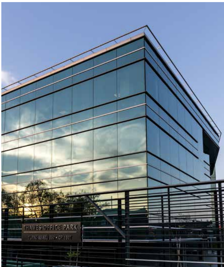
THAMES OFFICE PARK.
